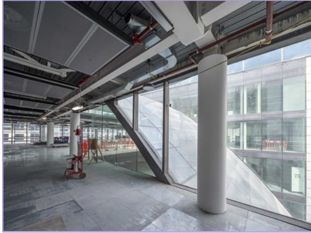
Level 6 CAT A Fit-out
