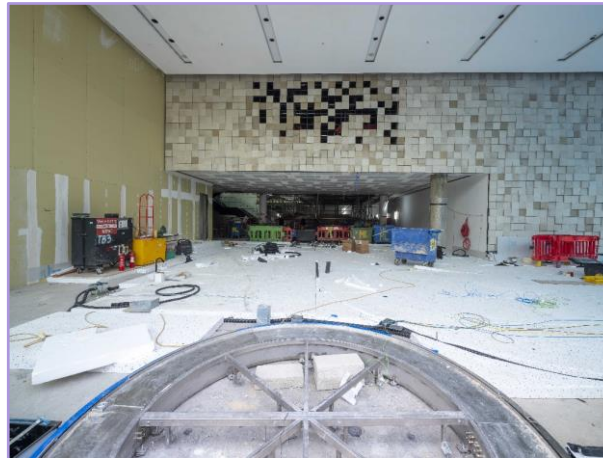
Front Entrance Reception
