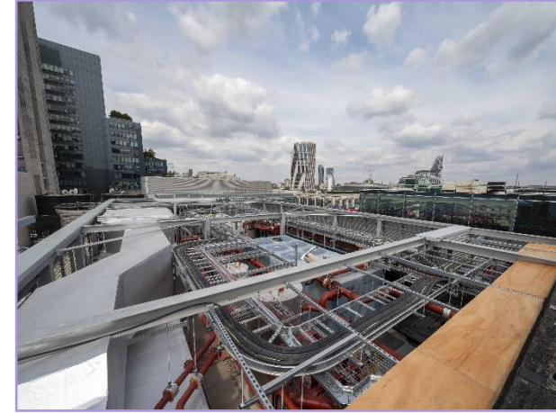
Roof Plant Enclosure
